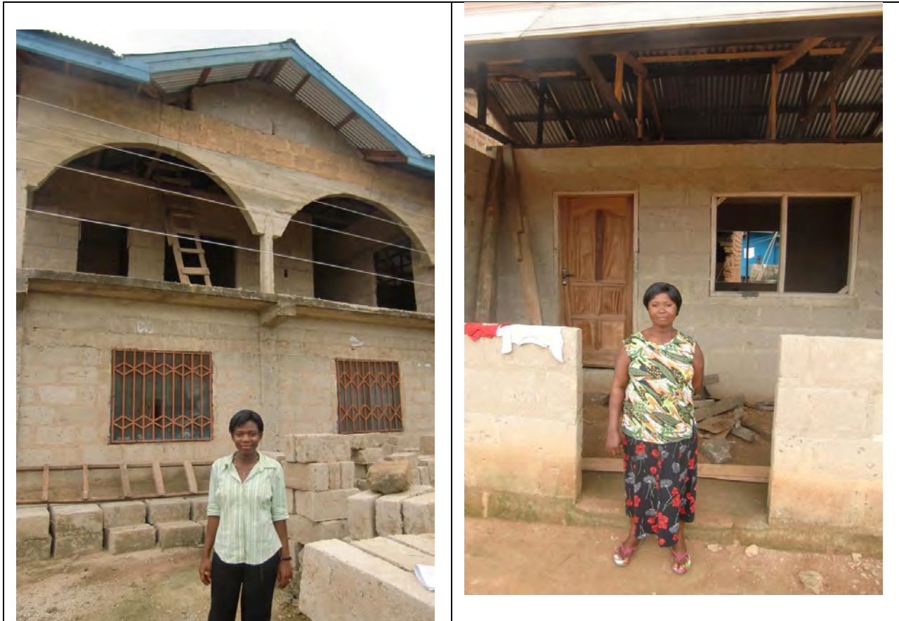
Of the 12 borrowers interviewed, four took loans primarily for roofing purposes and a fifth also took a multiple purpose loan that also included work on his roof. The unoccupied house on the left is owned by a household with two adult incomes, including waged employment from the husband. The woman on the right is the sole breadwinner in her family and plans to move in now that she has put a roof on her house which is constructed on land owned by her mother. This is the first individual loan she has ever taken in her own name.
