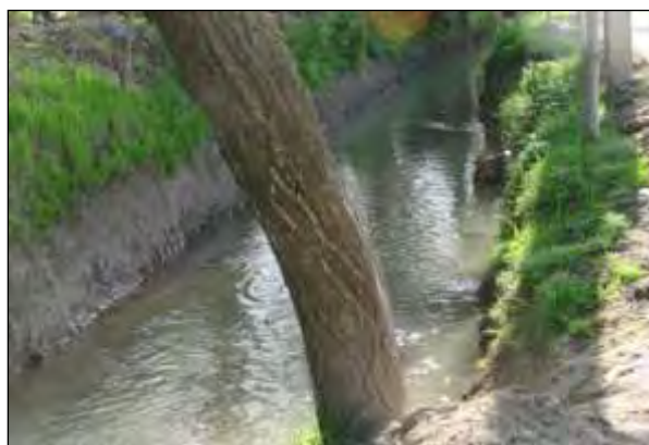
WUA “Juyi Mavloni” (Rudaki District) has a well-maintained irrigation canal.
