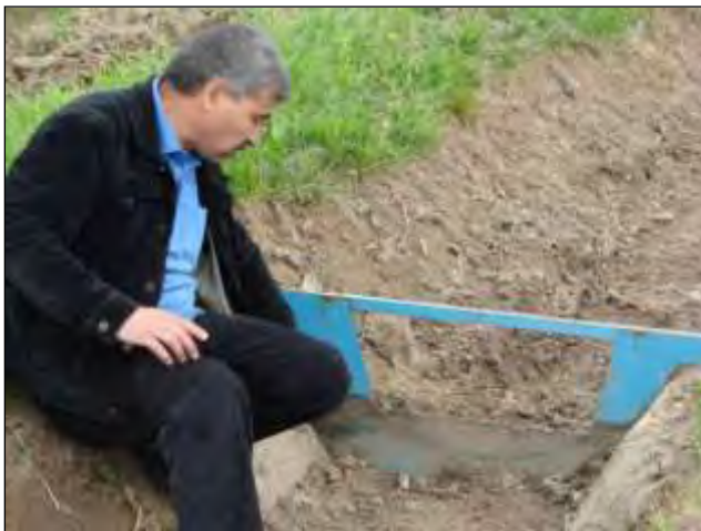
WUA “Shaynaki Gado” (Rudaki District) installs a new flow meter installed in a narrow canal.
