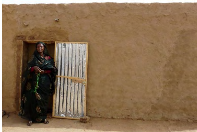
Figure 6: Fatima Mint in Trintame Village standing in front of her newly built home.
