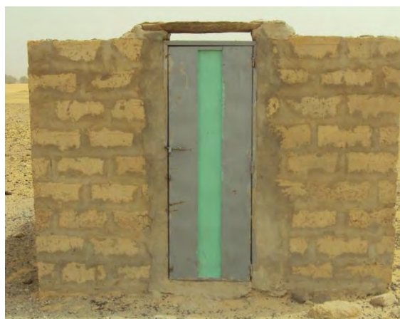
Figure 4: School latrine constructed in Medaine, Hodh el Gharbi with one door
