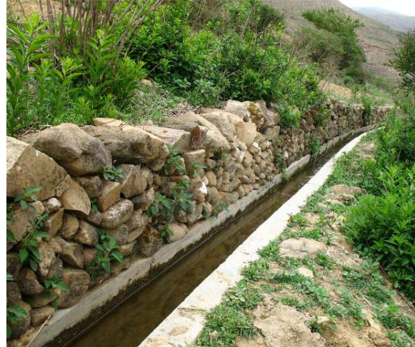
Mitigation, stone wall to retain soil.
