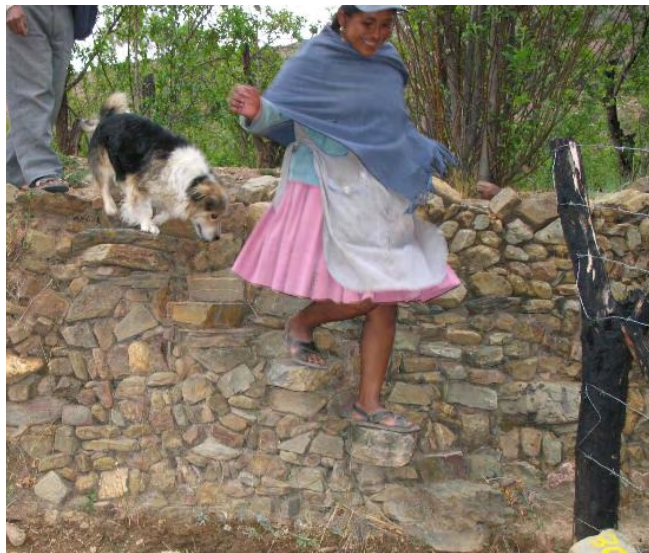
Walking down the stone steps built into the wall of a stone terrace. Note the thriving peach trees.
