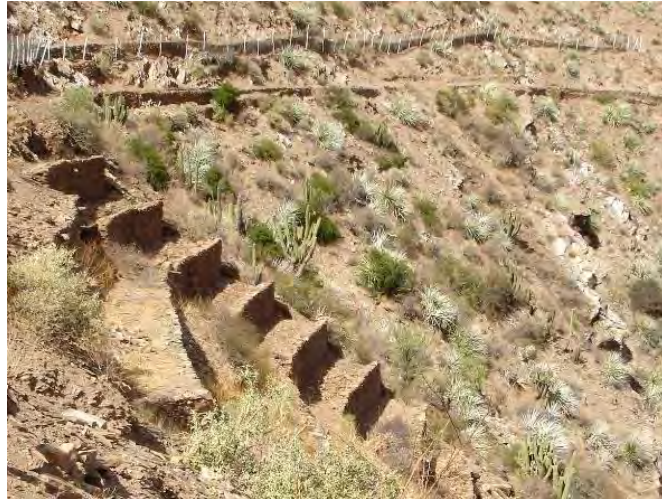
Newly built terraces ready to be filled with soil.
