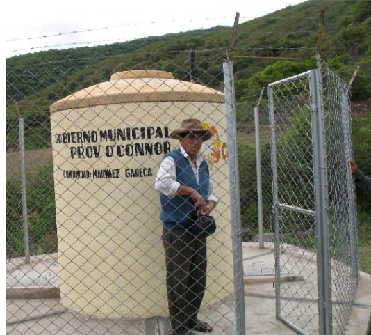
Ferro-cement water tank, safely locked and fenced. The municipal government is prominently named on the tank (along with CARE and USAID).
