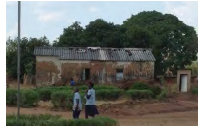
Staff housing in Nyimba District, Zambia
