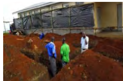
Operating theatre before renovation, Kyenjojo District, Uganda
