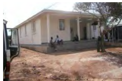
Operating theatre after renovation, Kyenjojo District, Uganda
