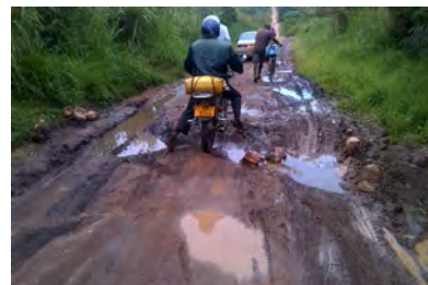
Flooded road in Kamwenge District, Uganda
