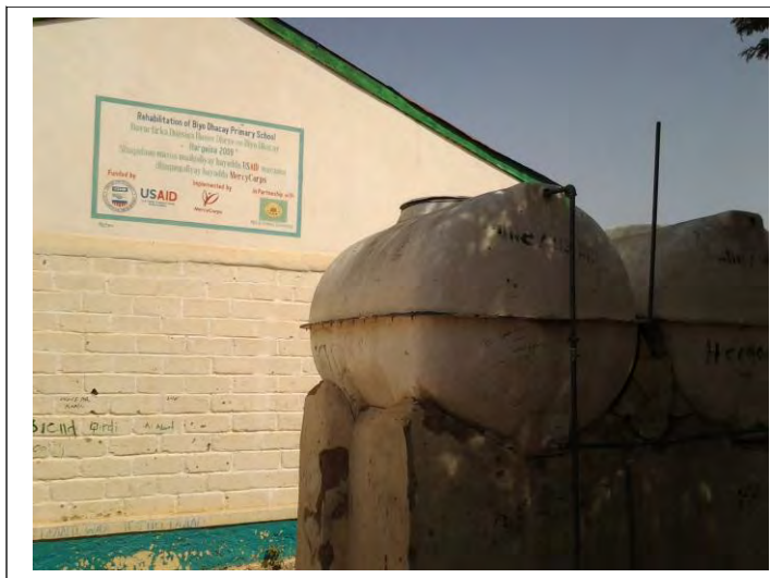
A classroom and water tanks constructed by SEEDS Program
