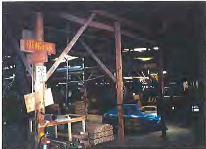
Placing translucent panels in the roof will reduce electricity demand.
