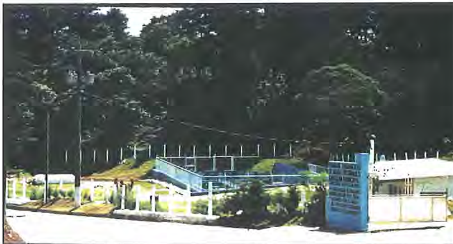
The sewage treatment plant in Fraijanes.
