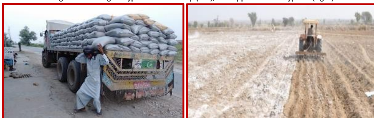
Image 3 Unloading of Gypsum at ASP Shop (left); Soil Application of Gypsum (right)
