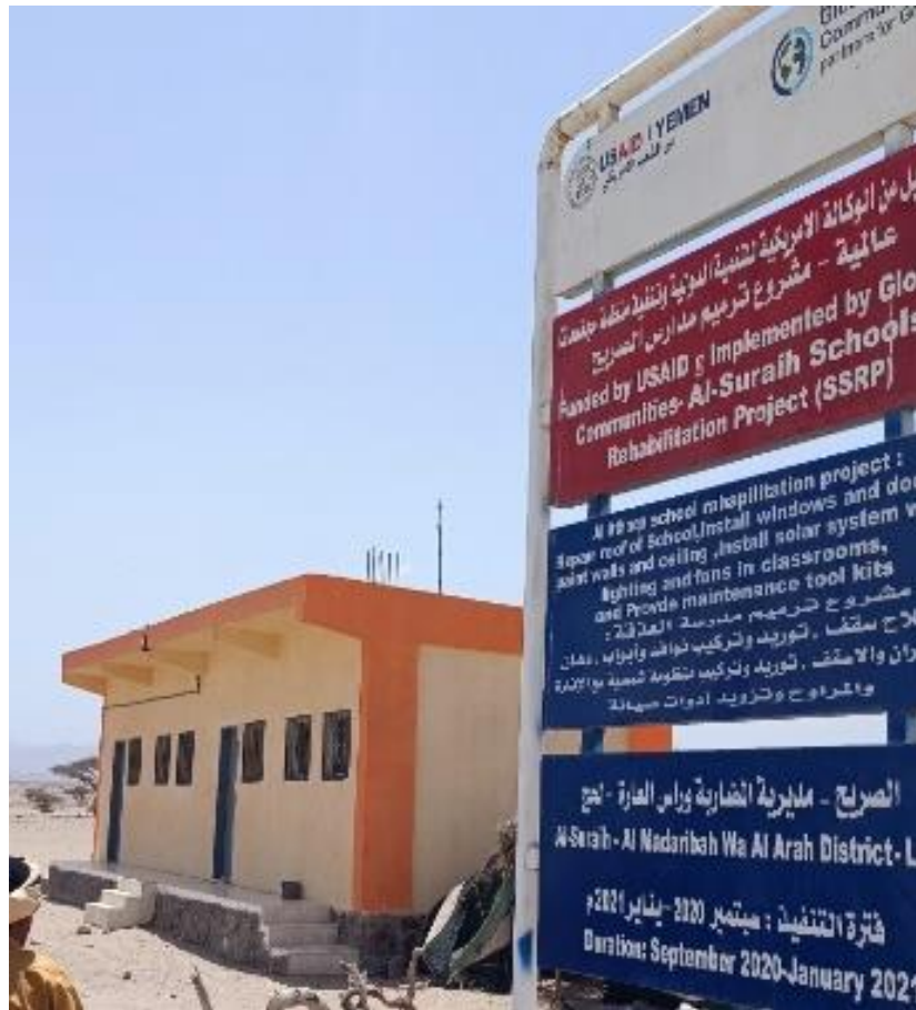
Al Sharaj School Rehabilitation Project
