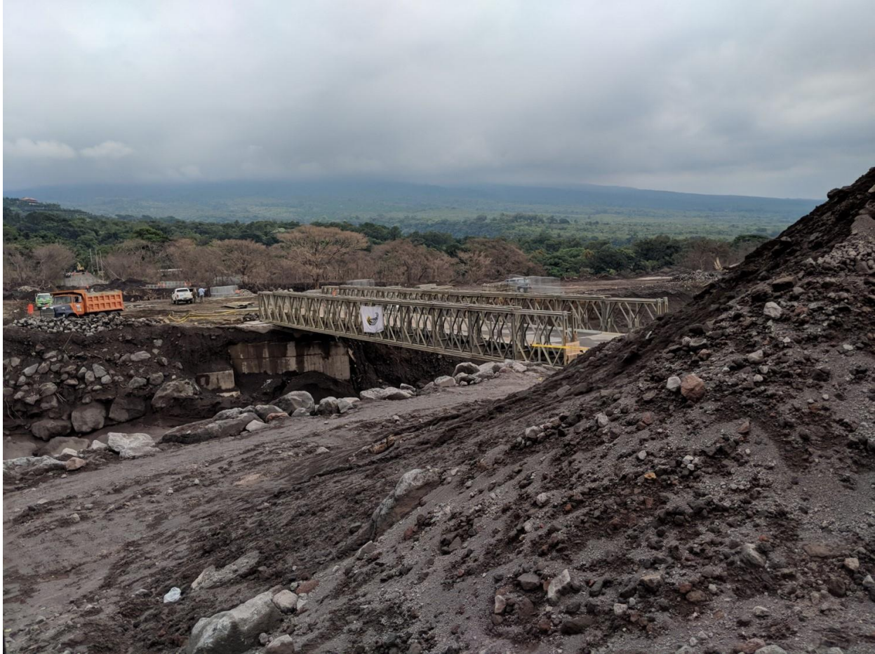
Temporary bridge constructed over Rio Achiguate drainage affected by pyroclastic flows and subsequent lahars from Fuego in Guatemala.
