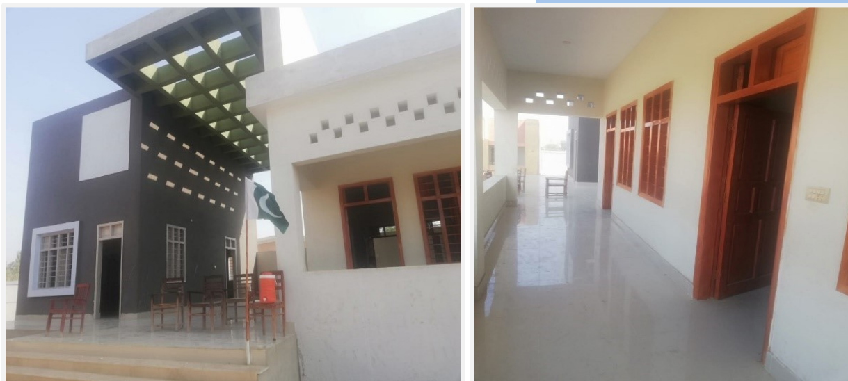
Two repaired/renovated school buildings in Larkana district.
