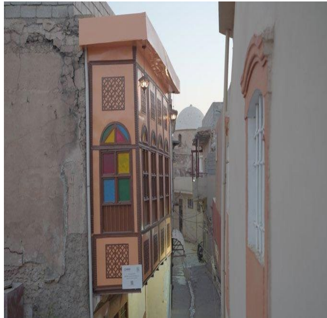
A "shanasheel" in the Old City of Mosul, restored with IRP I support.
