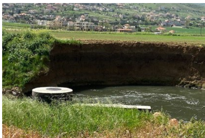
Figure 4. Rehabilitated intake from Litani River to the Khirbet Qanafar Wetland
