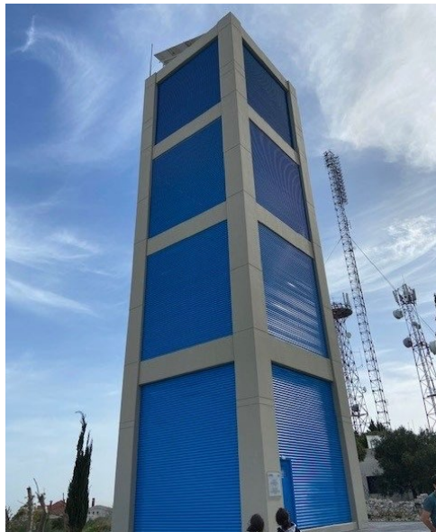
Figure 2. Qalhat elevated reservoir in Koura DA
