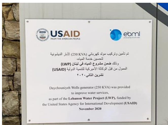
Figure 3. Generator installed by LWP in Deychouniyeh wells
