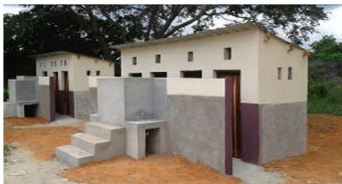
Figure 10: New blocks of latrines built at Sapala
