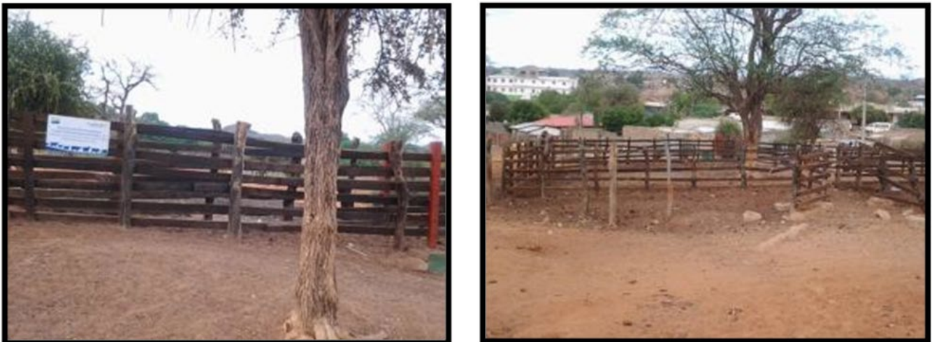
FIGURE 34: THE NEWLY REHABILITATED NGUNI LIVESTOCK MARKET LOADING RAMP AND ASSEMBLY BAY
