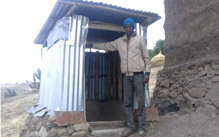
Figure 2 Better quality latrine Constructed.
