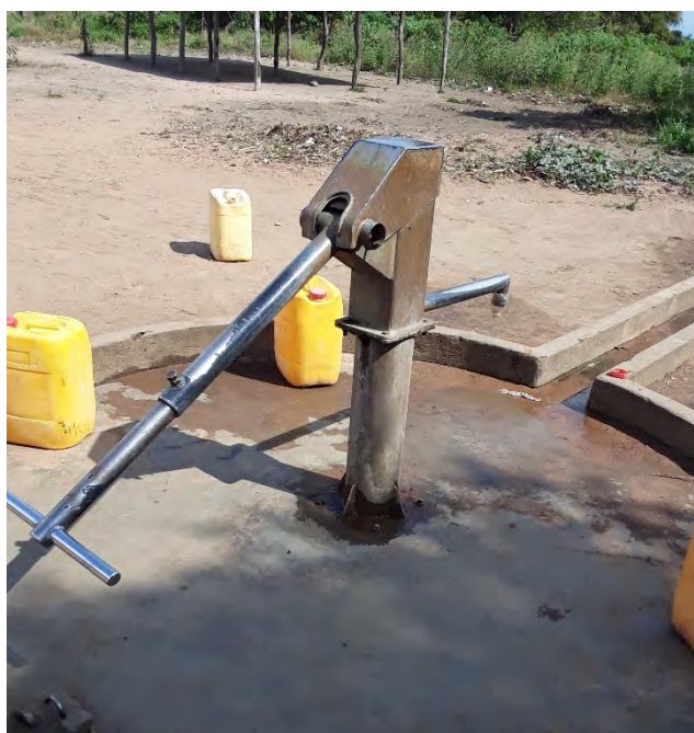
Figure 3: AFRIDEV Water Point Constructed Through SCIP
