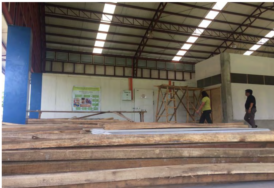
Figure 2. Cold storage facility inside the mango packing area (Carmen Mango Processing and Marketing Center)
