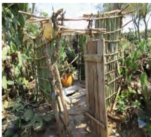
Figure 8. A Latrine with a Washable Slab and Tippy Tap in Anosy, Madagascar
