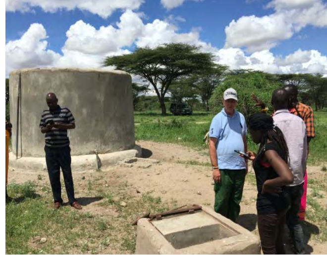
Figure 7: Human Wildlife Conflict in Nakuprat -Goku, and elephant destroyed water installation
