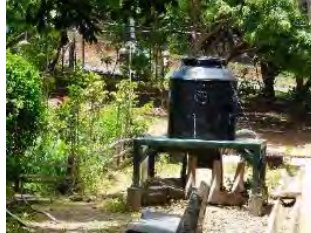
Photo 11 Improved water fountain. Escuela Rubén Darío El Sauce, León. June 2019
