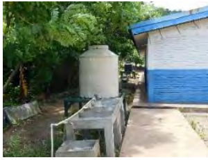
Photo 10 F Improved water fountain at the Flor de Sacuanjoche School, San Nicolás, Estelí. June 2019
