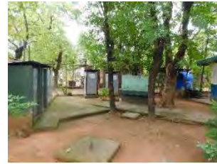
Photo 12 Improved latrine modules, San Juan School. Achuapa, León. June 2019
