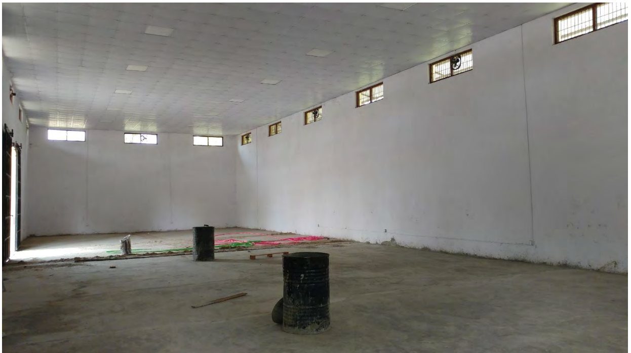
On-going construction at the “model” warehouse at Pathlaiya.
