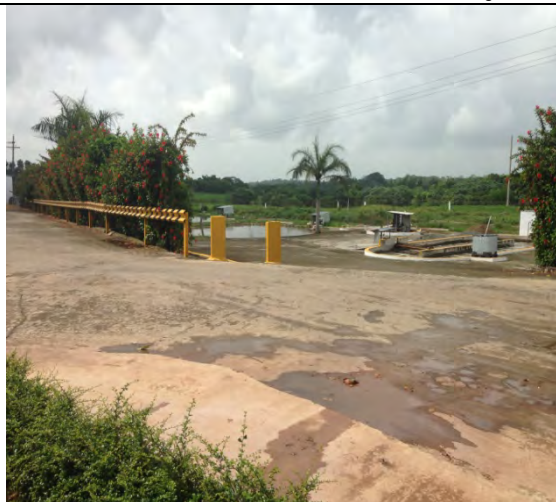
Figure 21. Plant wastewater treatment at the Alonso slaughterhouse
