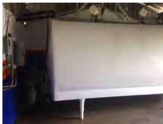
Figure 12 - Storage tank in one-tank MCC
