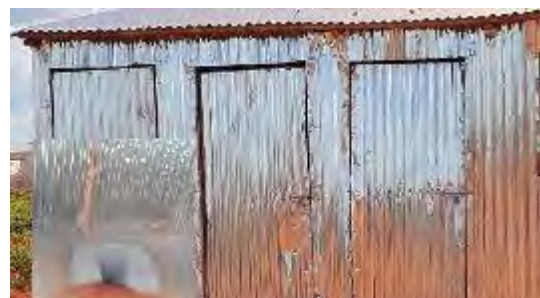
Figure 9: partial view of public toilets constructed by the project
