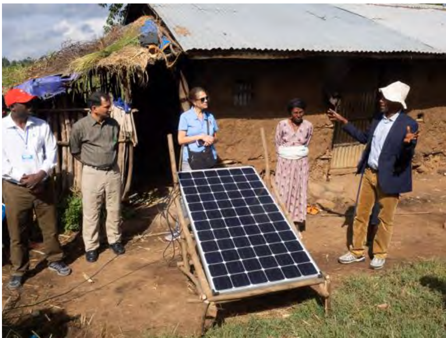
This solar panel is used to power the Magipump for water lifting
