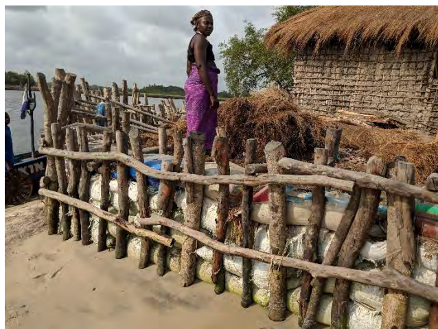
Figure 13: Momaya embankment at low tide
