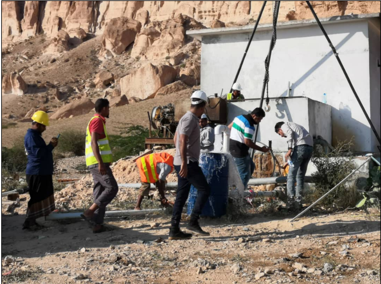
WATER PUMPING TEST CONDUCTED IN AL MAHFAD COMMUNITY, ABYAN GOVERNORATE
