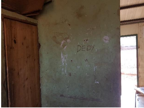
Malawi: Nkomadri School, adobe brick partition, Image by IMC staff, 2018
