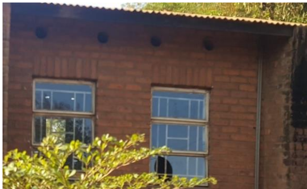
Malawi: Nkomadri, passive ventilation (conventional), Image by IMC staff, 2018
