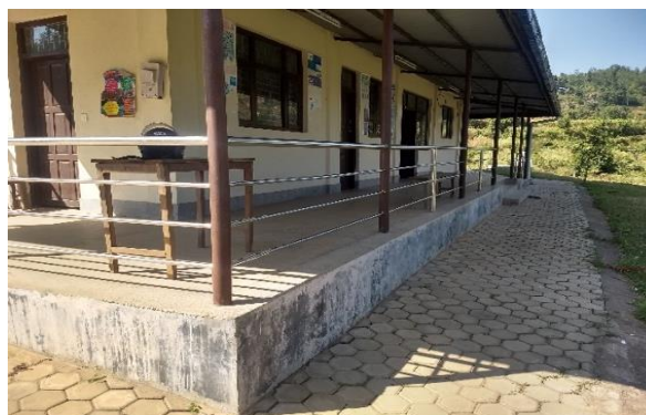
Nepal: Khoplang Health Post heavy doors (conventional), Image by IMC staff, 2018
