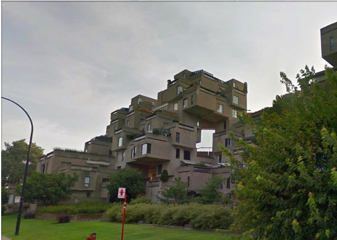
Habitat 67, Montreal, Quebec, CN (Screen Capture via Google Earth 2018)
