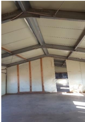
Malawi: Tsbango I Schools, substantial metal structure (prefab), Image by IMC staff 2018
