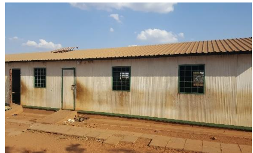
Malawi: Sire School, facility observed in good condition (prefab), Image by IMC staff, 2018
