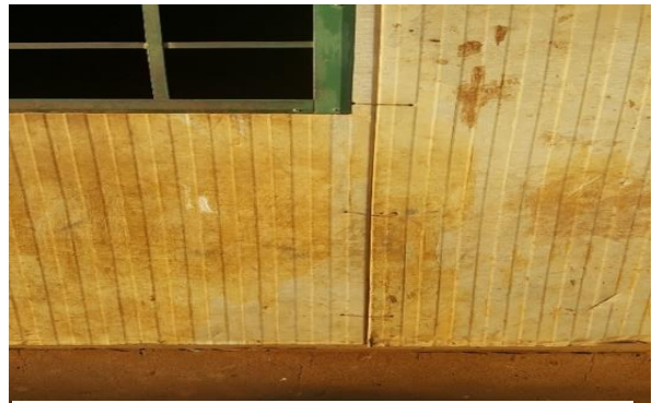
Malawi, metal wire fasteners at damaged panels (prefab), Image by IMC staff, 2018
