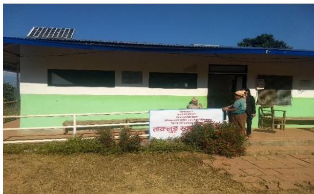
Nepal: Opportunity Village, partial roof collapse (prefab), Image by IMC staff, 2018
