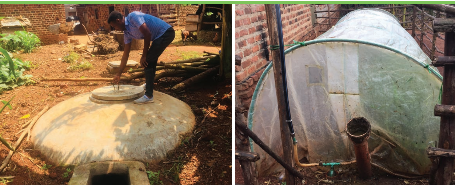
Fixed Dome type (left). Flexible Balloon type (right).
