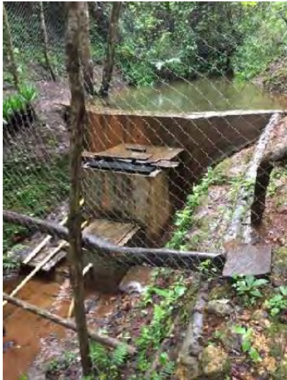
Water Intake for Treatment Watershed 6: Community of Puerta del Ocote
