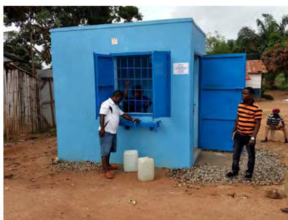
Figure 5: Standard USAID Water Vending Kiosk in Voinjama.
