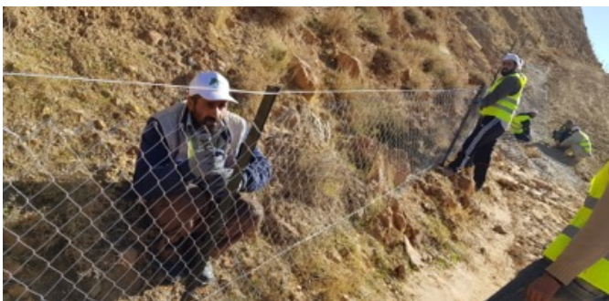
Figure 5. Daily workers installing a fence on a former quarry site to protect recently planted trees
