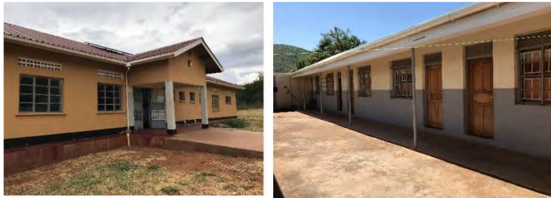
Examples of GHG health infrastructures, maternity ward and student lodge, Kaabong
