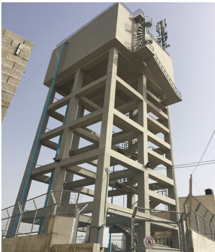
3Construction of a Water Reservoir, Rantis, West Bank
