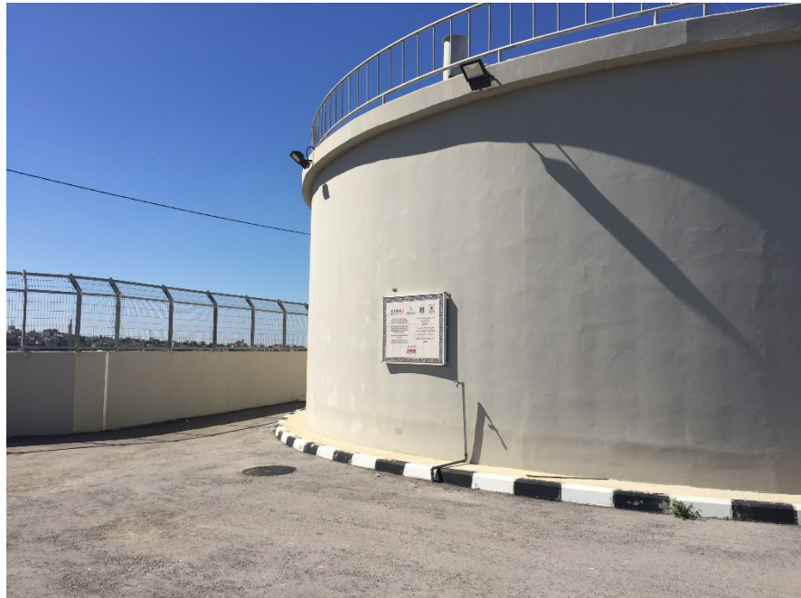
Water Reservoir and installation of main water lines, Attil, West Bank
