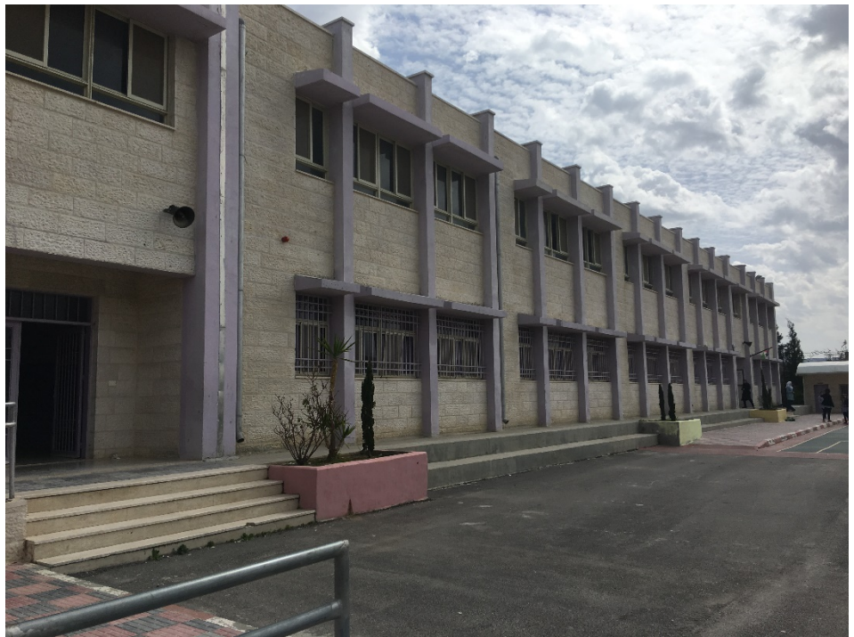
2 Construction of additional rooms and external works, Secondary School for Girls, Bil'in
