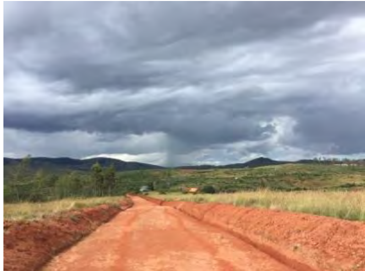
Road constructed under Food for Work
