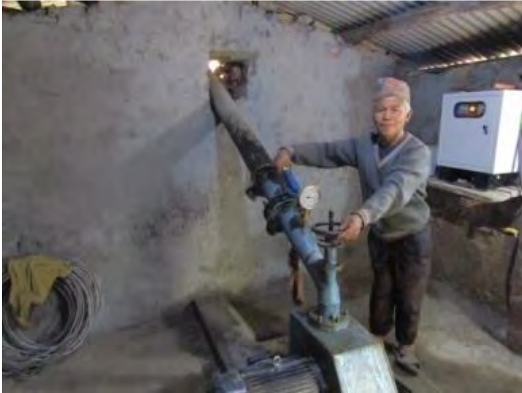
Plate 11 Rehabilitation of Balphe Rangrung Khola Micro Hydro Project
