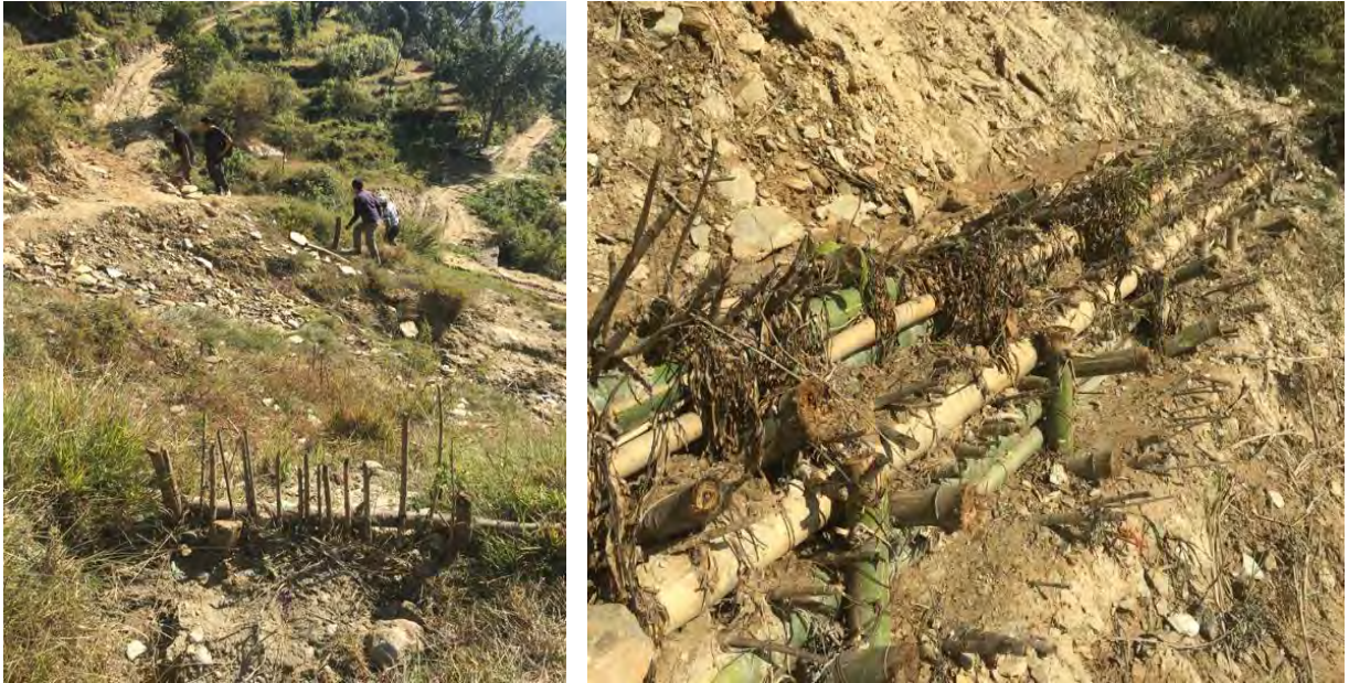
Plate 12: Bioengineering using crib walls and allied techniques
