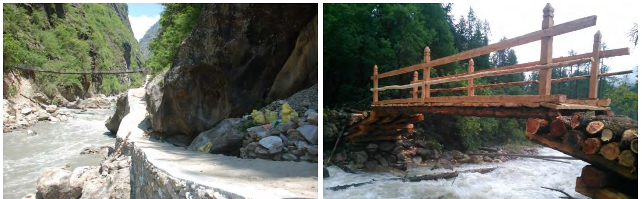
Plate 8 Trail improvement at Nyakphedi and wooden bridge reconstruction on Rubinala trekking trail
