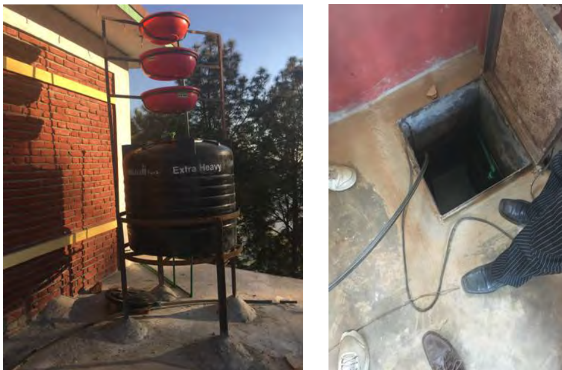
Plate 15: Water tank and aeration project (WASH Program)
