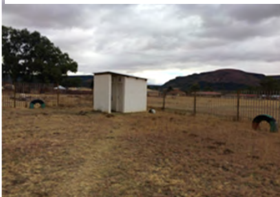
Figure 32: Toilet Facilities at the CMR Site
