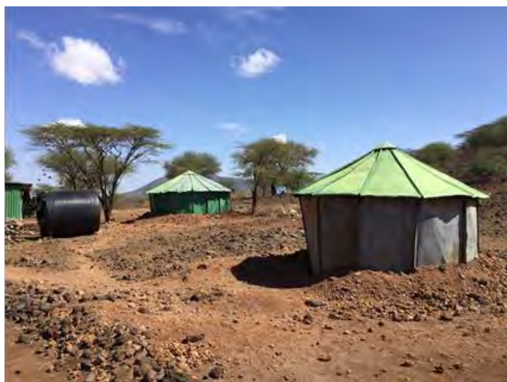
Community rangers' quarters, Namunyak conservancy, Samburu County.
