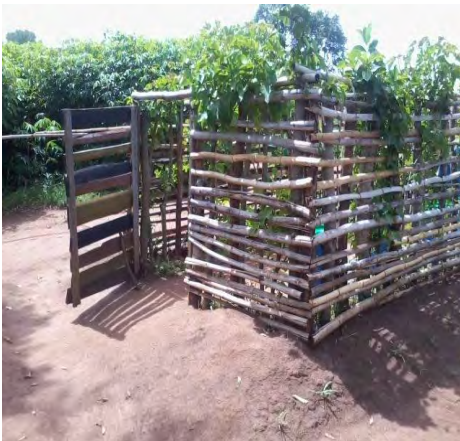
Photo 2: IRS wash areas and soak pits are properly fenced off to prevent public access
