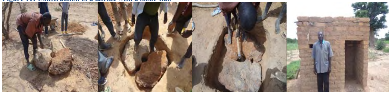
Figure 10: Construction of a latrine with a stone slab
