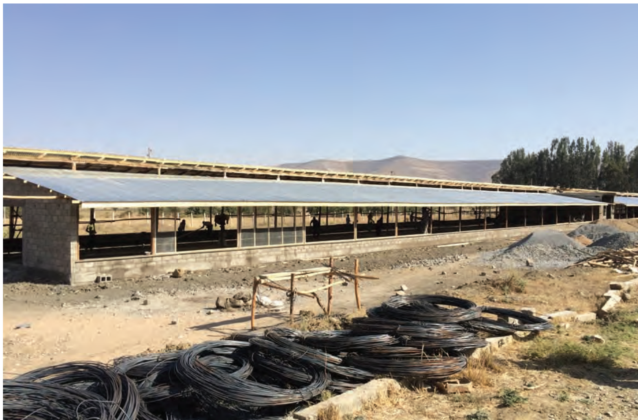
Construction of a new hatchery buildings from loan proceeds.
