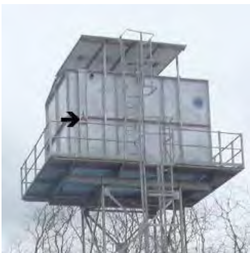
Figure 3: Mupoi PHCC reservoir. Arrow shows water level gage
