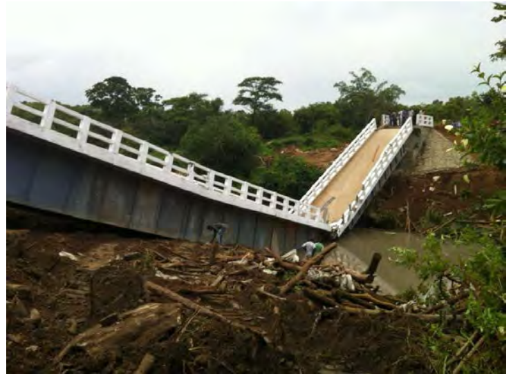
Figure 5: Kaya Bridge Collapsed Before Inauguration
