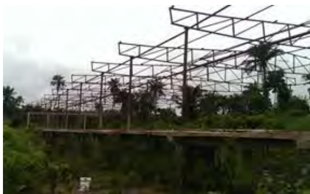
Site 2: partially constructed chicken houses
